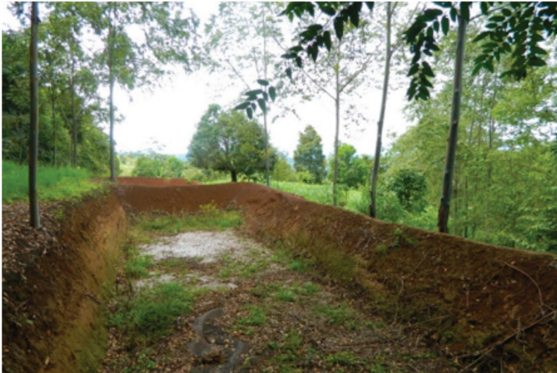
Figure 25. Water impounding pond (Location: Claveria, Misamis Oriental).
